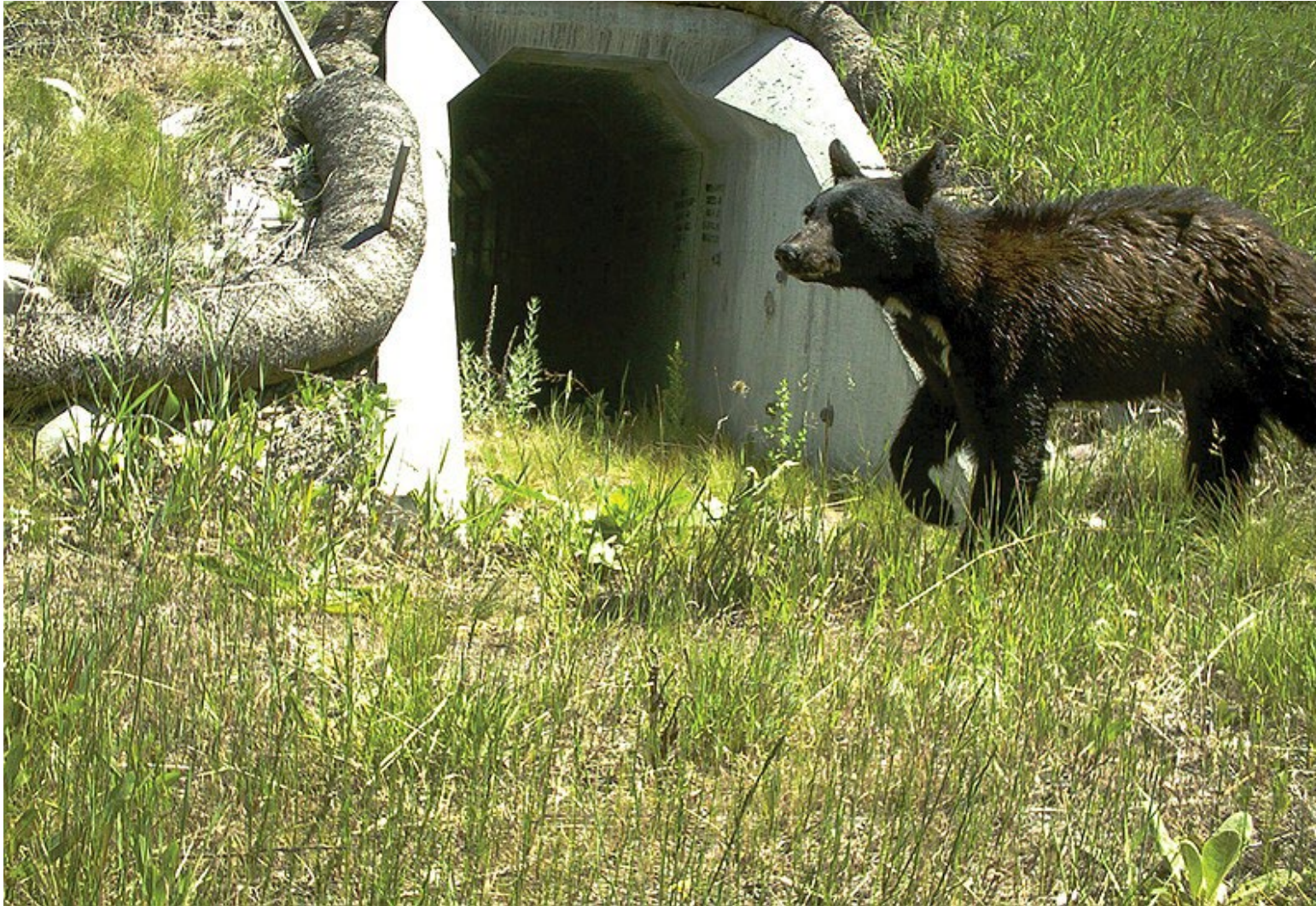
Example of a wildlife crossing along I-40 in the Smokies region
